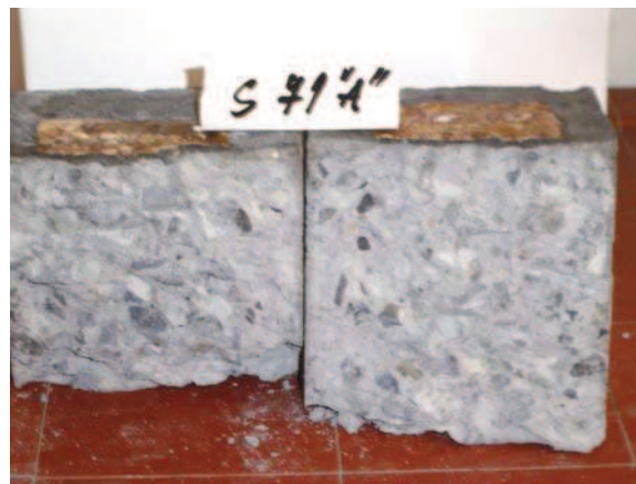
Fig. 5. Correctly composed mix, uniform distribution of the aggregate.
