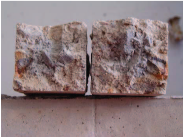
Fig. 13. Character of the geopolymers concrete after firing.
